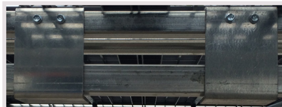
Anti-Tip Brackets to be Mounted on 1" Square Anti-Tip Bracket Crossbar
